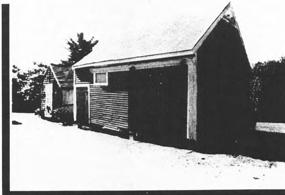
A8 - View of Shed From Northeast
