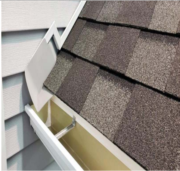
Kick out flashing with vinyl siding_134447.jpg
